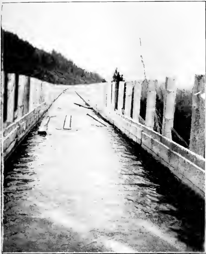
SHOWING FLUME CONSTRUCTION.
